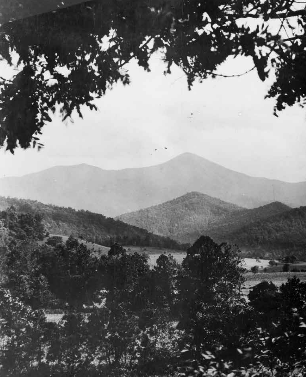
The Densely wooded Pisgah Forest, where men of the 328th Labor Battalion were sent to rebuild and repair logging roads in June 1918.
