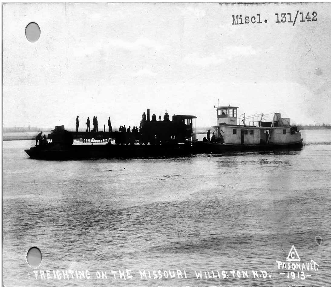
Above: In the absence of bridges, steamboats ferried railroad engines and cars across the rivers, as shown in this photograph from Williston, North Dakota, 1913. Record Group 77, Records of the Office of the Chief of Engineers.
