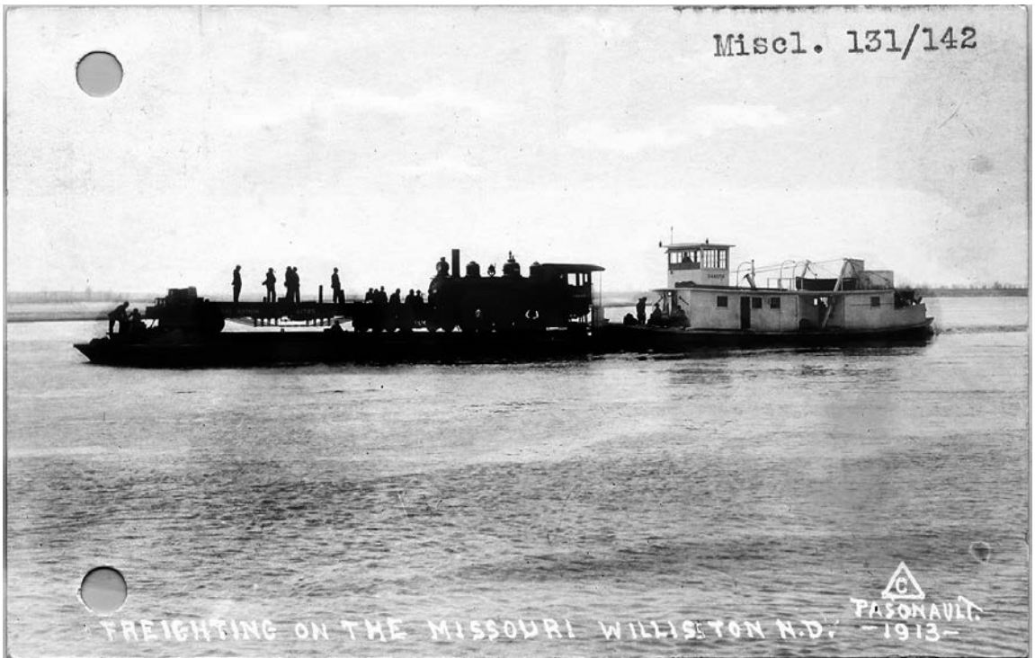
Above: In the absence of bridges, steamboats ferried railroad engines and cars across the rivers, as shown in the photograph from Williston, North Dakota, 1913. Record Group 77, Records of the Office of the Chief of Engineers.
