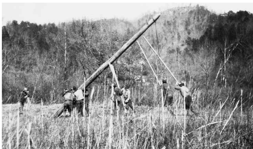
Left: A map of the Eastern Band of Cherokee Indians Reservation, 1934, shows the towns of Wolf Town and Yellow Hill, roads, locations of towers and telephone lines, and sites where Eastern Band members worked on CCC-Indian Division projects, marked in red spots. Above: Workers raise a pole on the Cherokee Soco telephone line.
