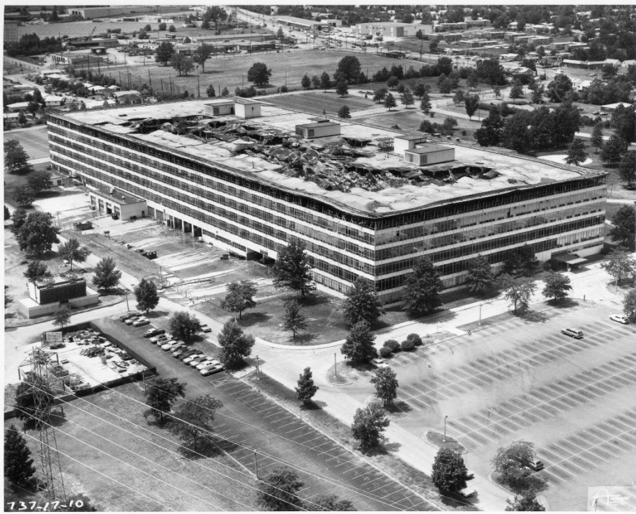
Left: Aerial view of collapsed roof Center: Warped shelving and piles of wet, charred records Right: Collapsed roof with visible shelving
