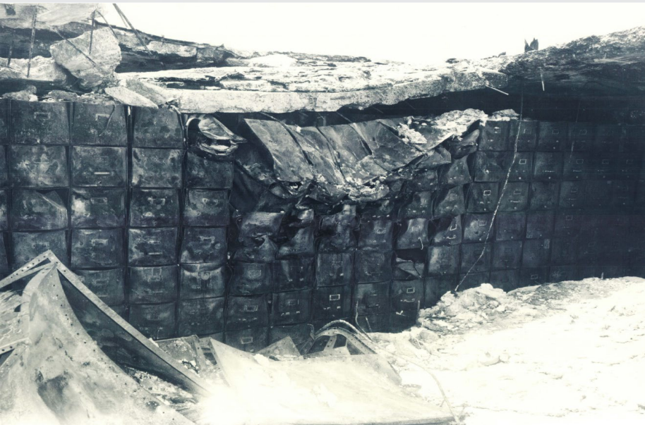
Melted steel filing cabinets used for record storage.
