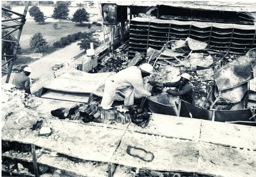
Workers attempting to salvage burned records and fragments from the floor and shelves prior to shelves being removed. They had to race to keep ahead of the clearance crew.
