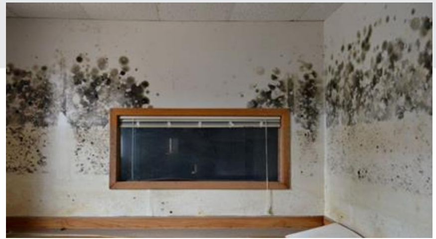
Minot, ND (2011). After high water flooding, mold grows on the walls of a local church. National Archives Identifier: 7856781 .
