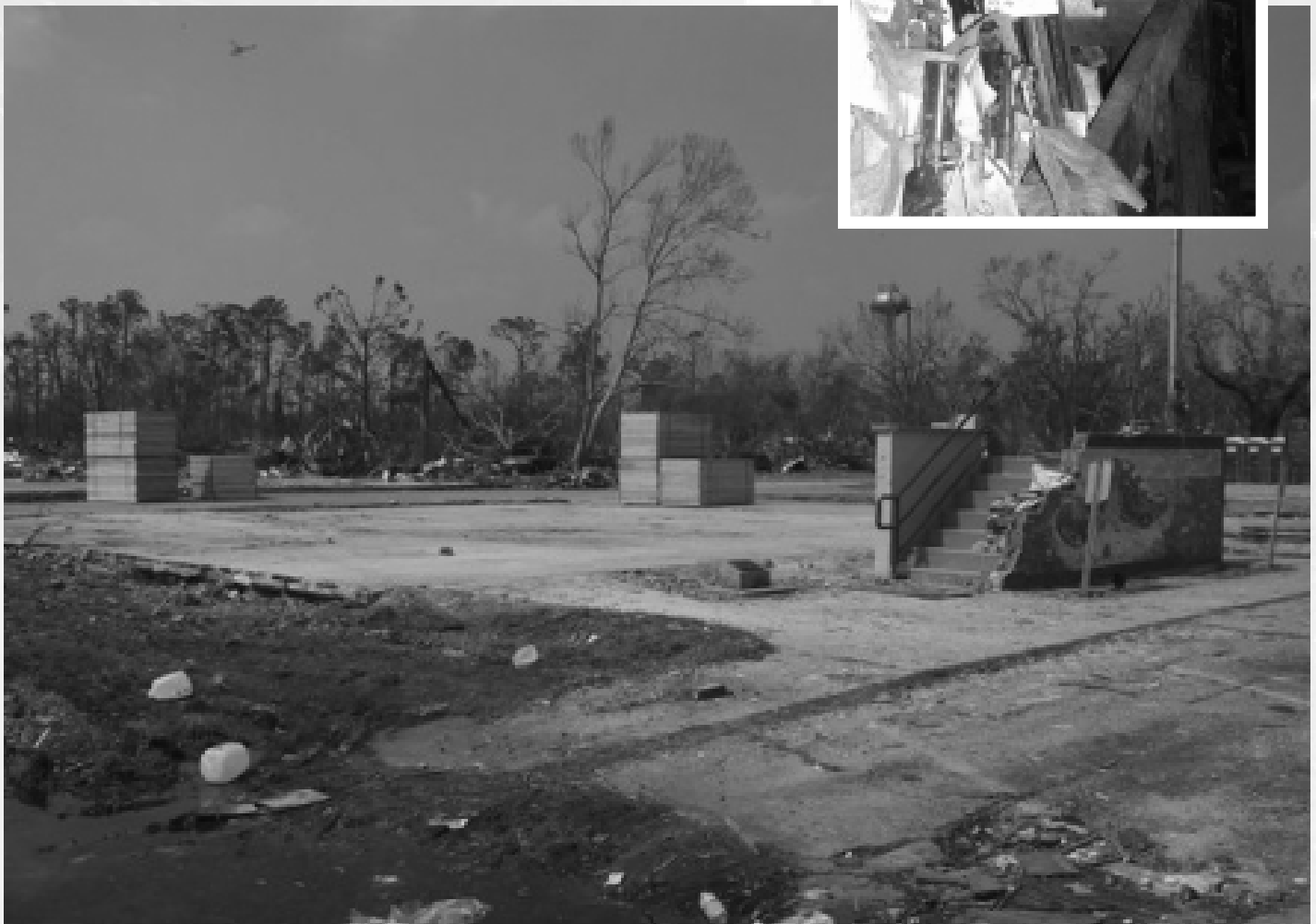
Remains of Waveland (Mississippi) City Hall. Photo: David Carmichael.
