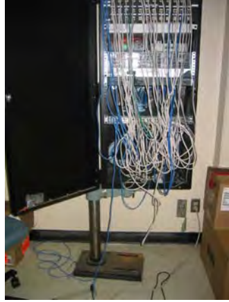
Figure 4. Jack needed to hold rack in place
