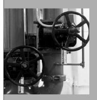
o achieve fire protection for the archival records stored at Archives II, a unique systems interface was developed between the fire sprinkler system, fire detection and alarm system, and mobile compact shelving control system.
