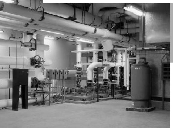
Pressure-reducing stations at various points in the building reduce the steam pressure from 110 pounds per square inch to 15 pounds per square inch for use in heat exchangers, heating coils, and some humidifiers.
