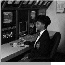
A 24-hour guard service protects the building and staff and monitors the security management system located in the security control room. The console pictured here includes a security computer that monitors intrusion alarms and access, closedcircuit television monitors, a videotape recorder, and a master intercom station.
