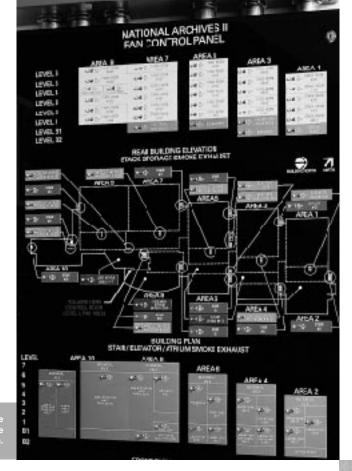
The fan control panel allows the fire department to manually control the smoke removal system.
