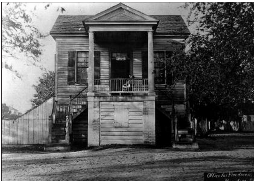
Most Freedmen came in contact with the Freedmen's Bureau at the local level such as at this office in Beaufort, South Carolina. (165-C-394)
