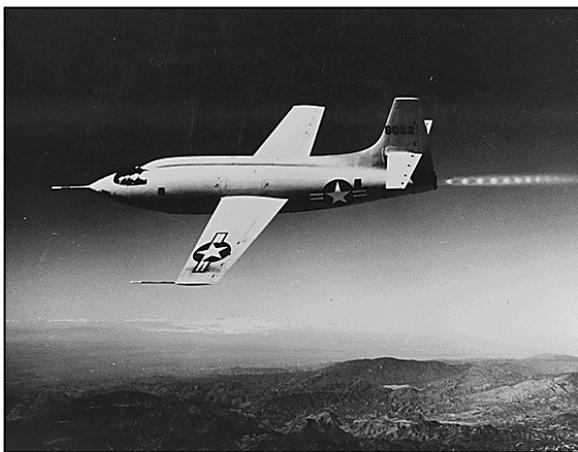
United States government to design and build advanced aircraft. The building and test flights of the experimental research aircraft, the procedures and personnel which established themselves on this project helped lay the foundation of America's space program in the 1960s. The X-1 project defined and solidified the post-war cooperative union between U.S. military needs, industrial capabilities, and research facilities.
